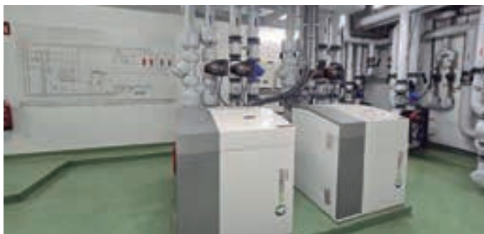
▲ Actual photographs of the installation
