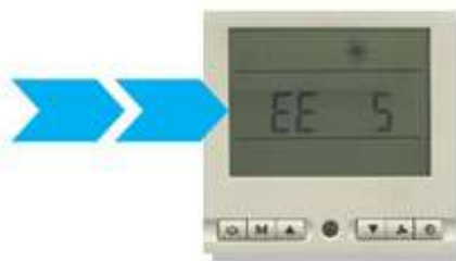
Error code ,EE5' advising of low / high water flow or damaged flow switch.
